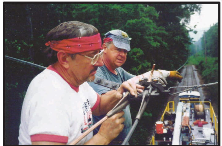
Above: Fred Walter with the late Phil Glass installing an overhead wire frog at Altoff siding in 1998.
