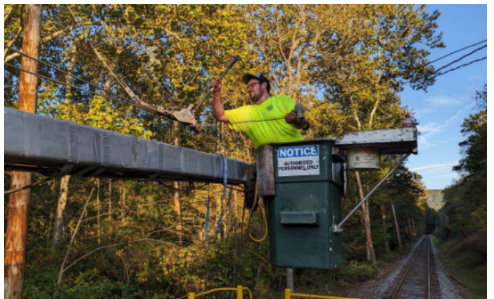
Below right: Nicholas Brightbill repairs overhead wire using the Aerial Bucket Lift Car.
